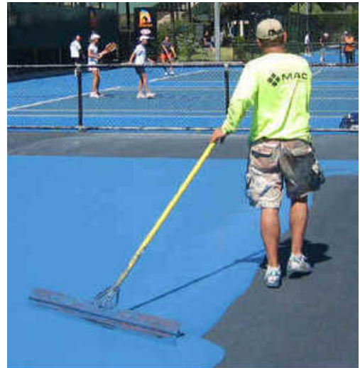
A McConnell & Associates employee helped work on the Plexicushion surface.
